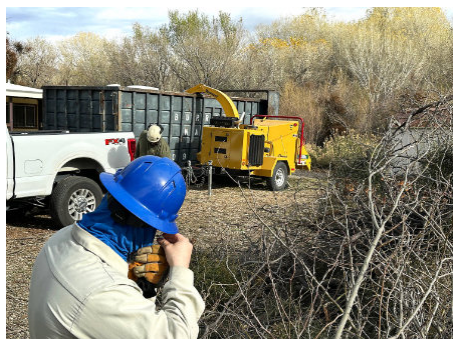
Work crews clear brush to help protect the Education Center from wildfires. BMCP photo.
